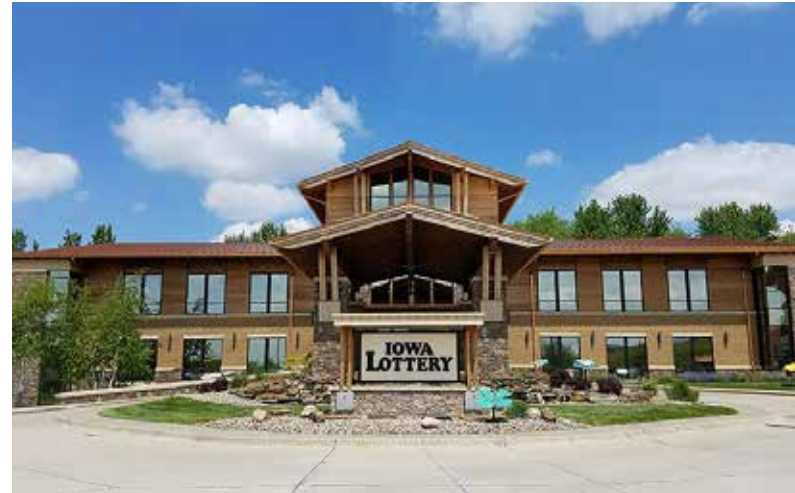
Iowa Lottery headquarters is located at 13001 University Avenue in Clive.
